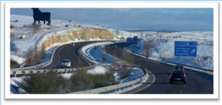
Figure 11.3. Overview of the A2 motorway.
