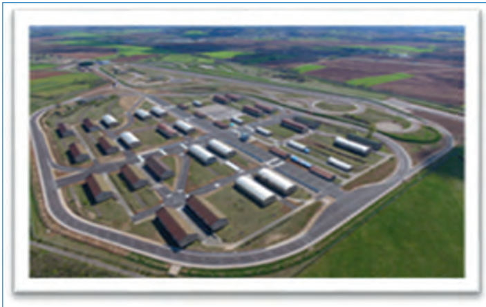
Figure 11.5. Aerial View of the Transpolis site.
