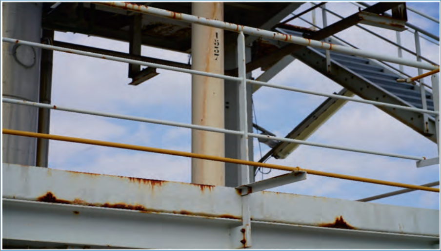
Figure 3.7. Sample image taken during the pilots for detecting corrosion in pipes.
