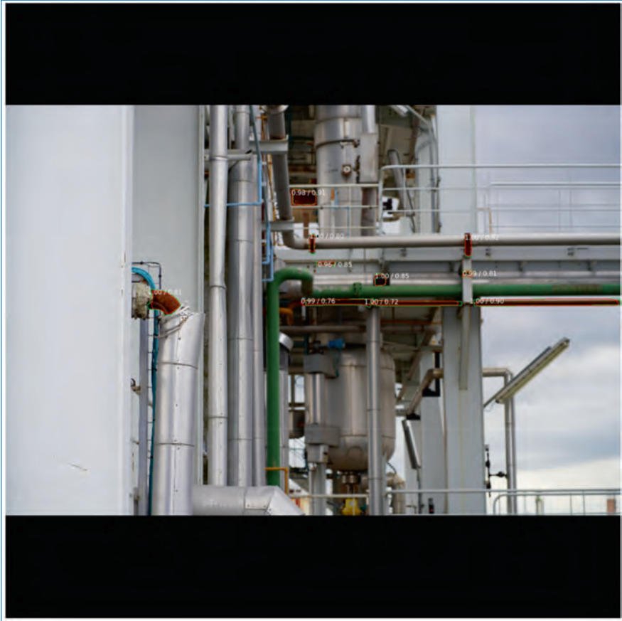
Figure 3.14. Sample image predictions on the test set using MaskRCNN. Green is the ground truth annotation, red is the prediction. Next to each annotation there is the confidence/IoU.
