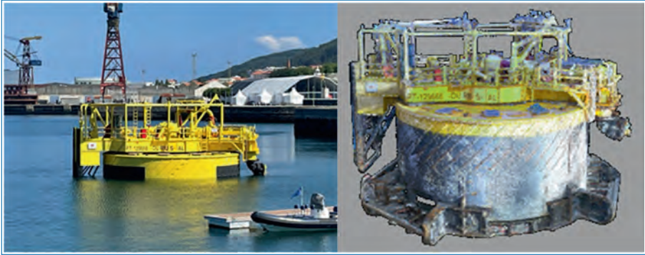
Figure 9.3. Floating Structure installed on the Coastal Testbed of the ATLANTIS Test Centre (left) and point cloud reconstruction (right).
