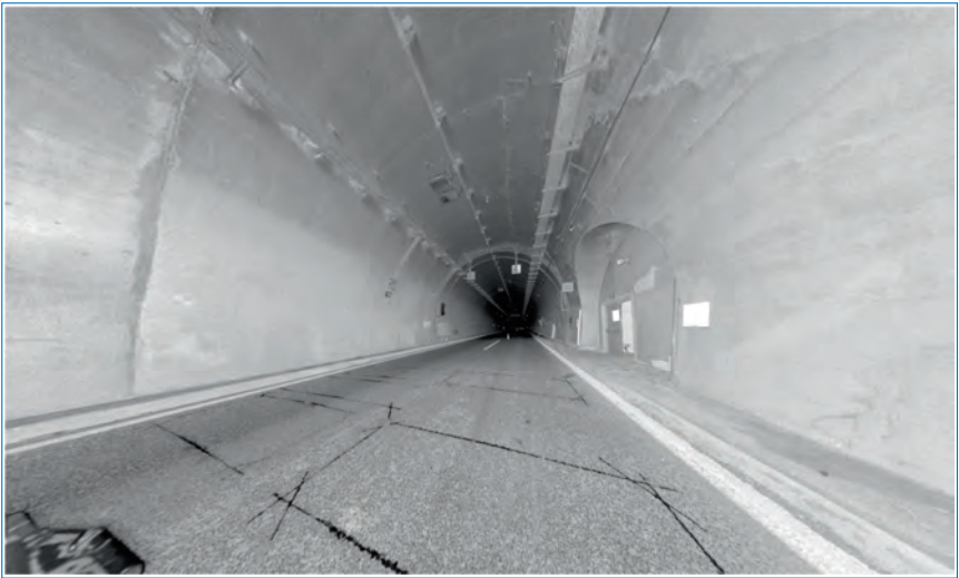
Figure 4.5. Tunnel 3D reconstruction (external view).
