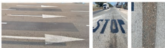
Figure 5. Left and Centre: Repainted signs with black paint; Right.: Continuous white line removed with pressurized water.
