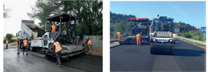
Figure 9. Paving and compaction detail of an asphalt mixture
