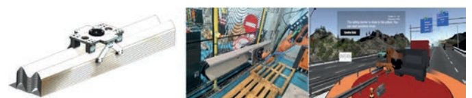
Figure 3. Left.: Attachment tool with the robotic arm; Centre: Robotic arm positioning the metal barrier; Right.: Virtual Reality for training operators in the installation of metal security barriers.
