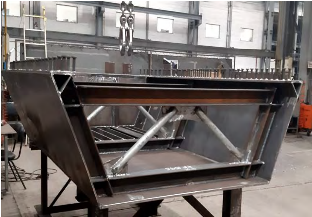
Figure 67. Steel structure of the box section
