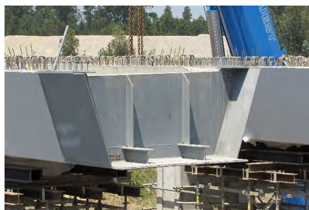
Figure 54. Connection piece (original design from PS35)
