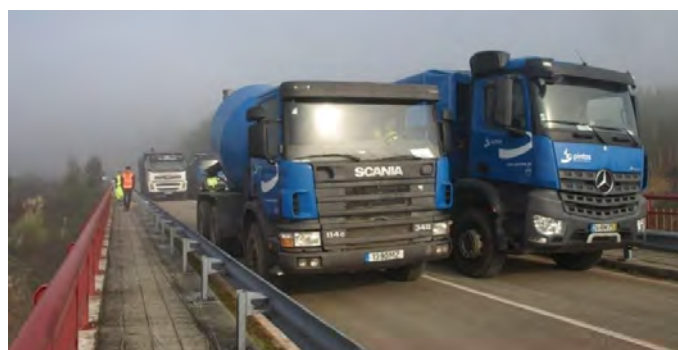
Figure 21. Trucks at the adjacent mid span (Load case 4)
