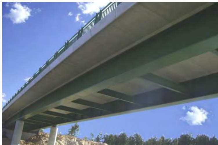
Figure 2. Steel-Concrete girders. Bottom view.
