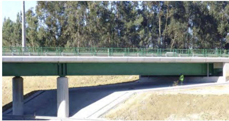
Figure 3. Steel-Concrete girders. Side view.
