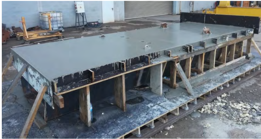
Figure 65. Freshly concreted upper deck slab
