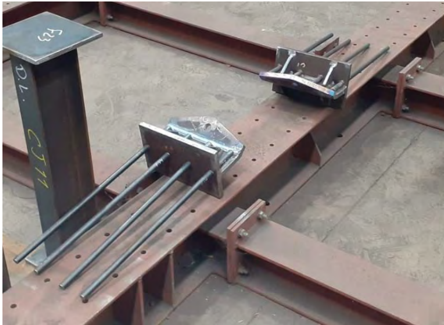
Figure 69. Suspension eyebolts with tie rods
