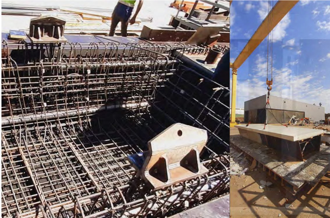
Figure 73 and Figure 74. Installing the eyebolts for prototype mobilization and weighing
