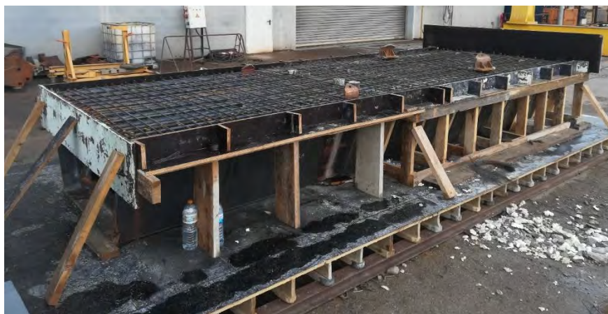
Figure 64. Formwork and reinforcement of the upper deck slab
