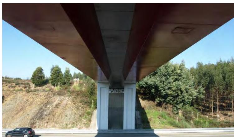
Figure 14. Bottom view of the overpass
