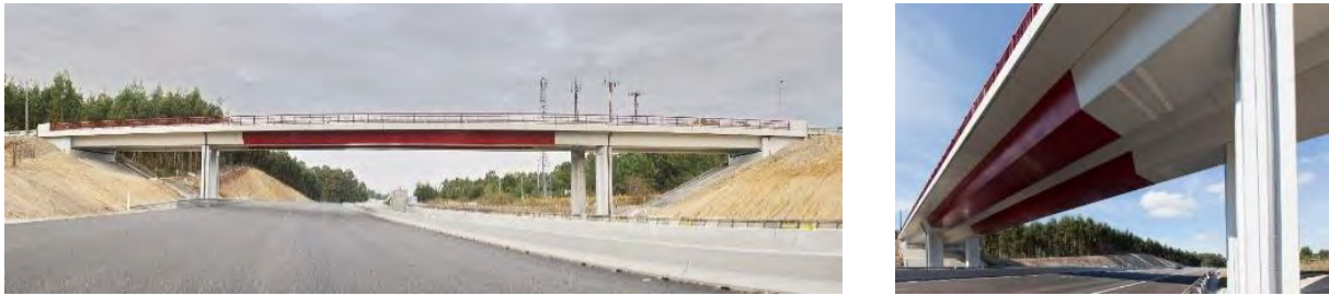
Figure 6. A Hybrid Bridge. Side and Bottom views.
