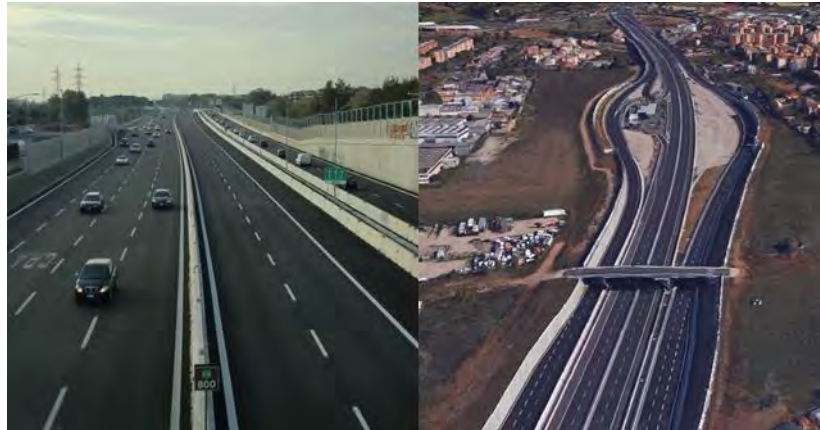
Figure 29. Urban segment of the A24 motorway – connection with Rome
