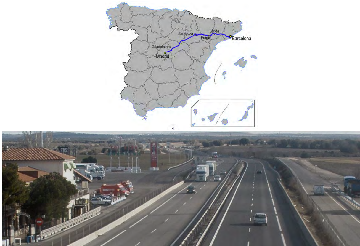
Figure 33. Localisation and overview of A2 (Reference: Acciona)
