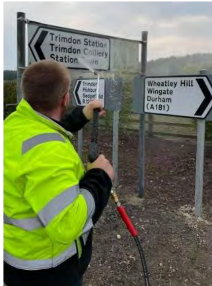
Figure 1 Road worker manually cleaning road signals
